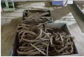
写真-1 杭切削時回収鉄筋
