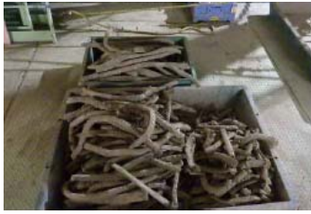
写真-1 杭切削時回収鉄筋
